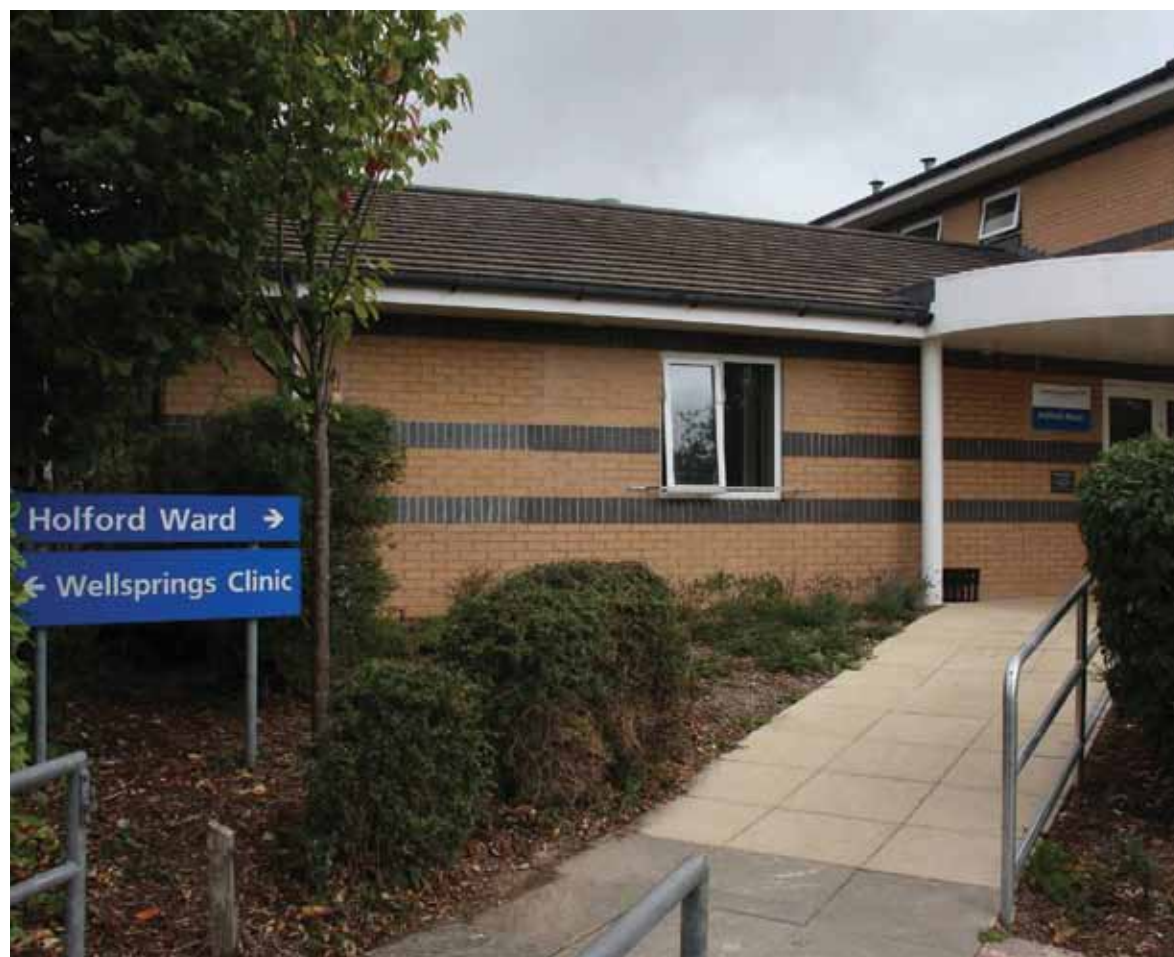
The restyled entrance to the refurbished Holford Ward, Taunton
