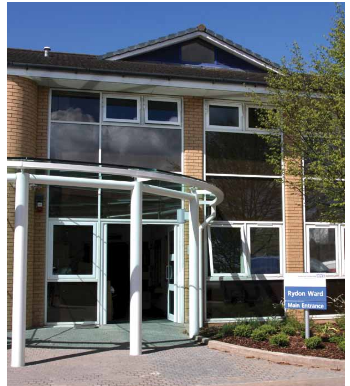
Entrance to refurbished Rydon Ward, Taunton
